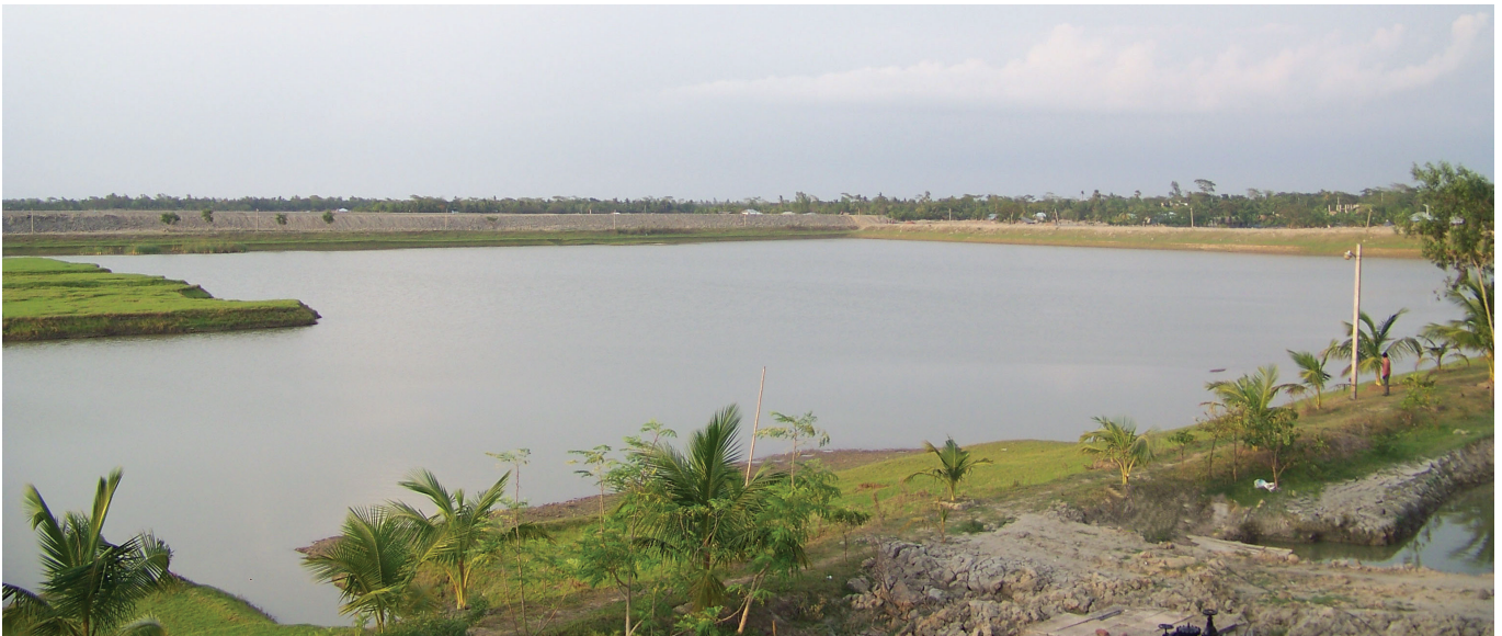
Rainwater harvesting in Mongla to provide drinking water to the city. © ICLEI South Asia
