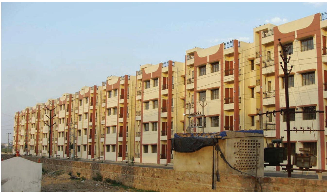
WELL EQUIPPED AFFORDABLE HOUSING WITH GOOD ACCESSIBILITY CAN ADDRESS MULTIPLE CONCERNS OF LOW INCOME GROUP
