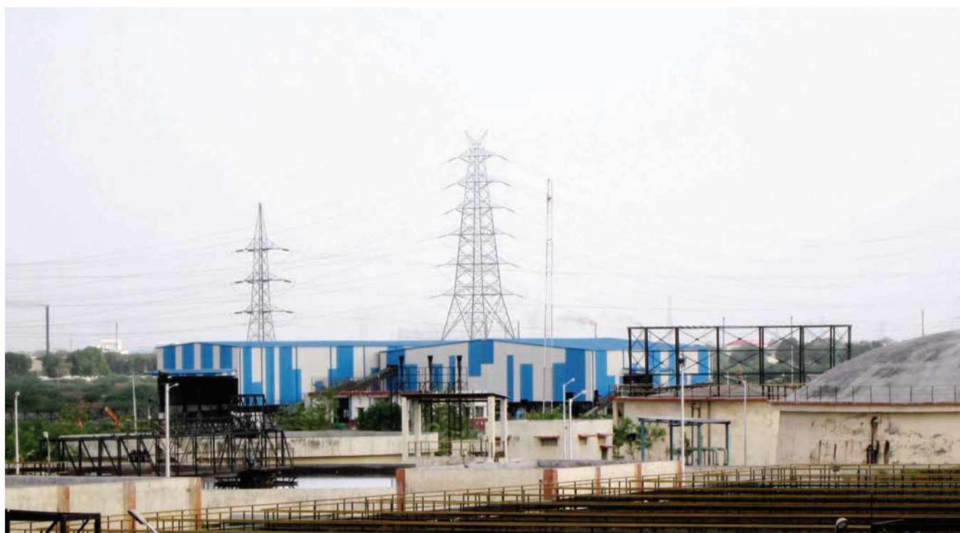
IMPROVED POWER TRANSMISSION AND DISTRIBUTION INFRASTRUCTURE CAN HELP TO MINIMISE POWER LOSSES
